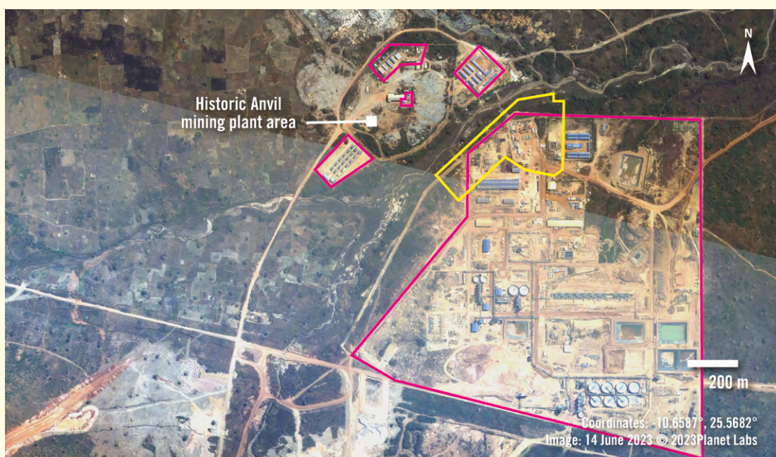
© ↑ Mukumbi, DRC: Satellite image from 14 June 2023, shows a recent image of the Mutoshi mining site. The old village area is highlighted with a yellow polygon, and the areas with new structures visible are highlighted with pink polygons. New structures are visible within the historic Anvil mining plant area.
